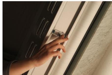
At this point the door is ready for operation. Run the panel up and down a few times to make sure no adjustments are needed.
