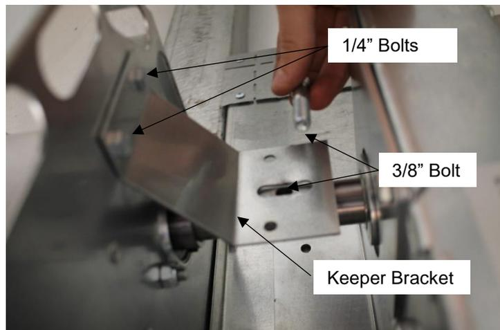
Install the chain keeper approximately 4' off the floor and 6" away from the side of the door track.
