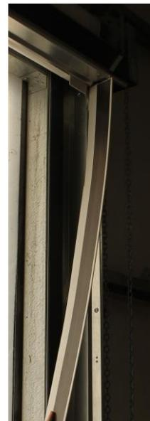
Rotate the front track toward the door opening 90 degrees a few times to make sure the front track moves freely.
