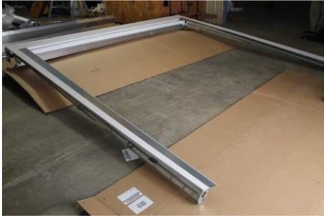
With the door frame lying face down and the tracks aligned with the frame opening, rotate the assembled frame upright by “walking” the legs upright as they are pinned against the cooler wall at the bottom.
