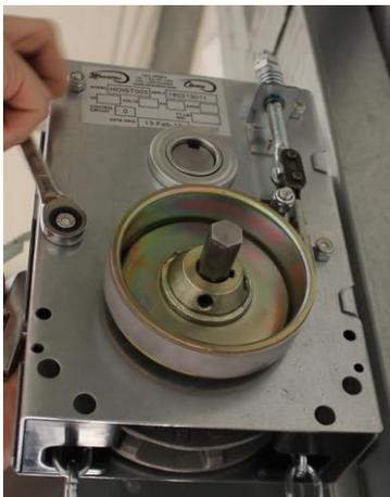
Position the hoist so that the four holes in hoist align with the four holes in the mount and insert the  $\frac{1}{4}$ "x3" bolts from the door hardware kit in these holes. They must be inserted from the mount side to keep from hitting the cover later. Use the four  $\frac{1}{4}$ " locknuts to tighten the hoist to the mount.
