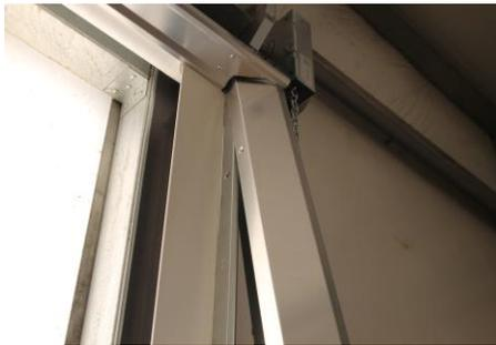
Take the right and left aluminum cladding pieces and attach them back to the door frame in the same manner they were removed. You will have to slide the top in first, lift up while pushing toward the door frame and slide the cladding down. Use the six phillips head screws that were removed before to re-attach the cladding.
