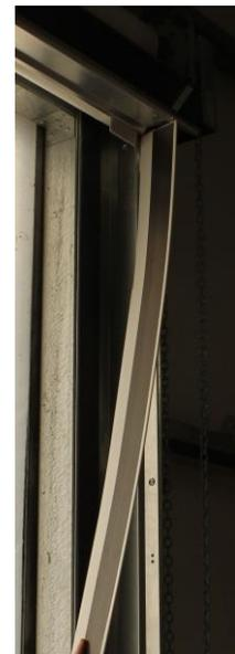
Rotate the front track toward the door opening 90 degrees a few times to make sure the front track moves freely.
